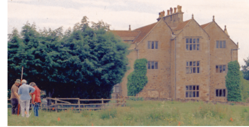
Gainford Hall, with the survey area in the foreground
