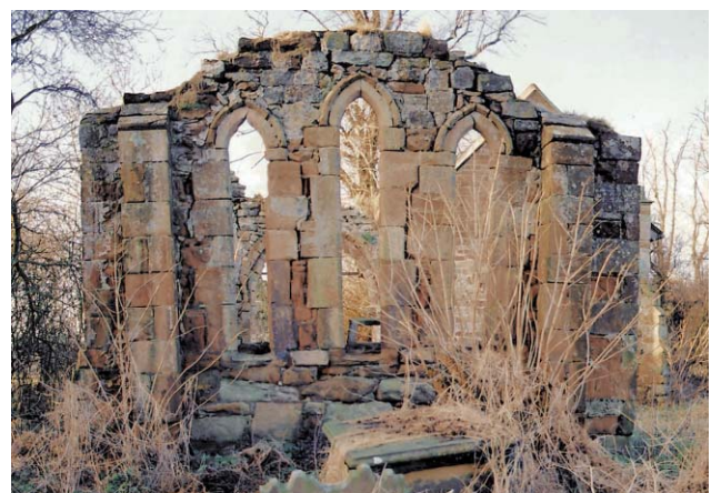
Sockburn Chapel, County Durham. © English Heritage
