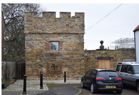
The restored tower and gate seen from Silver Street.
