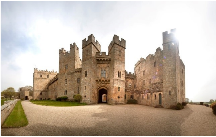
Raby Castle from the west. Four impressive towers can be seen from this perspective, from left to right; Clifford's Tower, the Watch Tower, Nevill's Gateway, and Joan's Tower. ©Peter Atkinson Photography.
