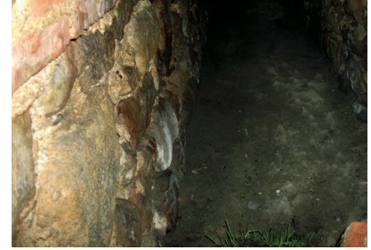
The brick-vaulted tunnel
